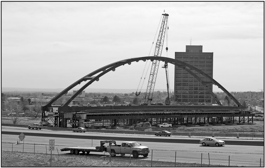
On March 18, 2010, this bridge was being assembled to span US Highway 6 east of Simms Street for the west corridor of Denver's light rail system. – Photo © 2010 Bruce Nall.
